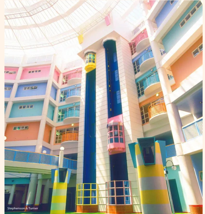
Stephenson & Turner. (2014). Starship Hospital . https://www10.aeccafe.com/blogs/arch-showcase/2014/11/20/starship-childrens-hospital-in-auckland-newzealand-by-stephenson-turner/
